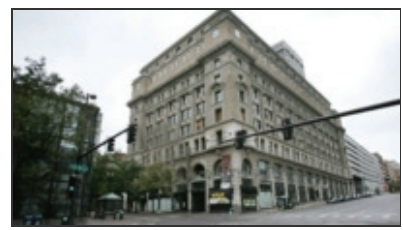
The Brandeis Building is located at 16th and Douglas Streets.
